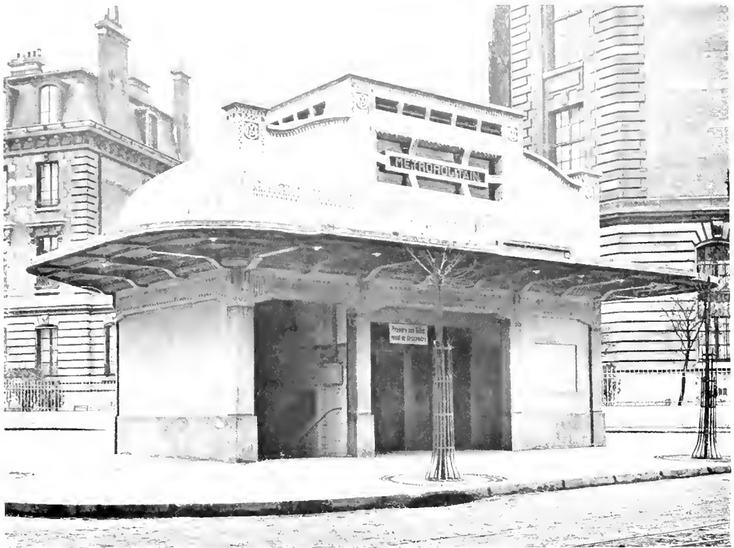
Station Pelleport : Façade principale.
